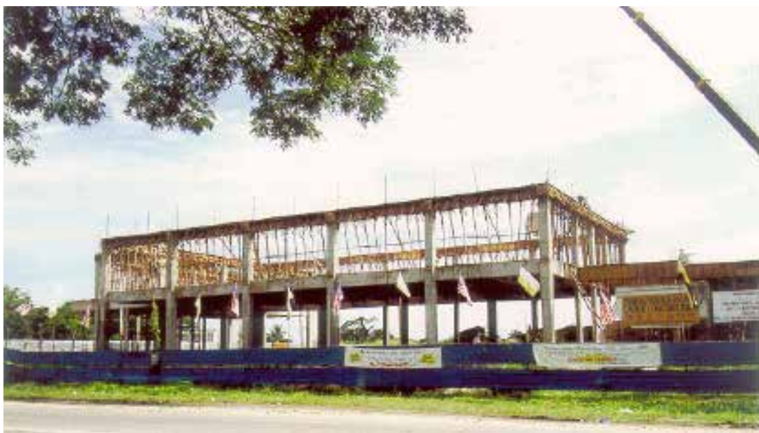
October 2005. Construction is Well Underway
