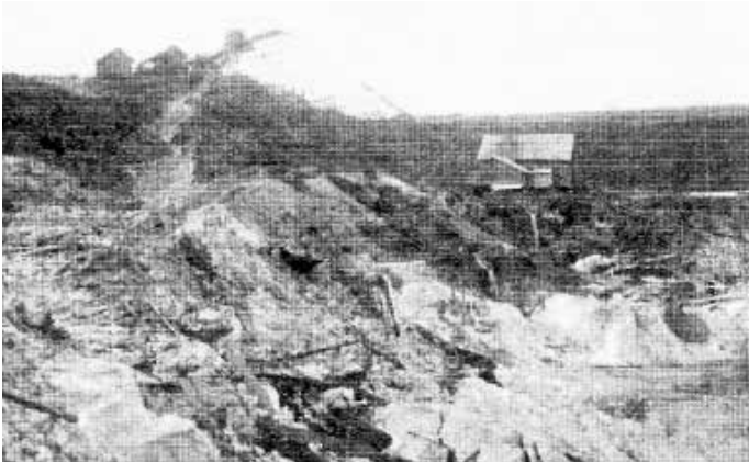
TWO STAGE GRAVEL PUMP MINE.
