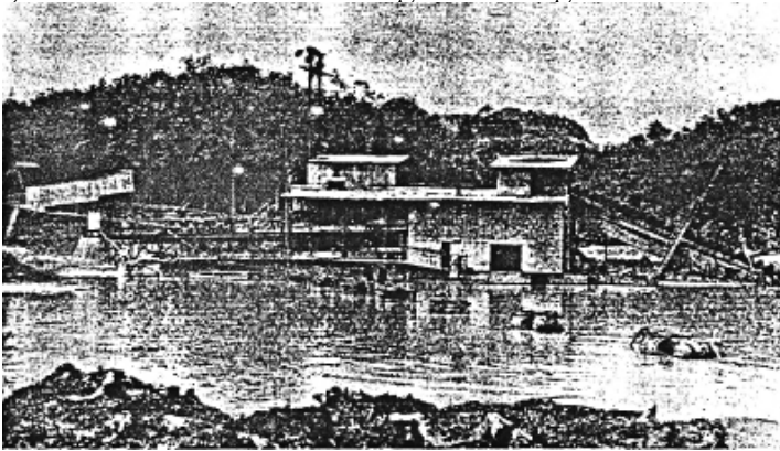
SPUD DREDGE WITH STACKER.
