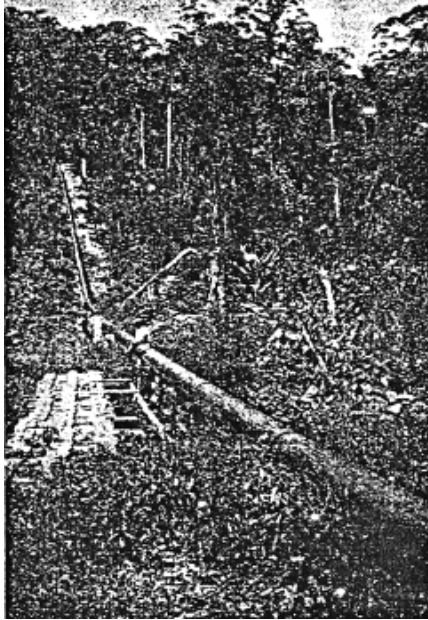
PIPE LINE CONVEYING WATER TO MINE.
