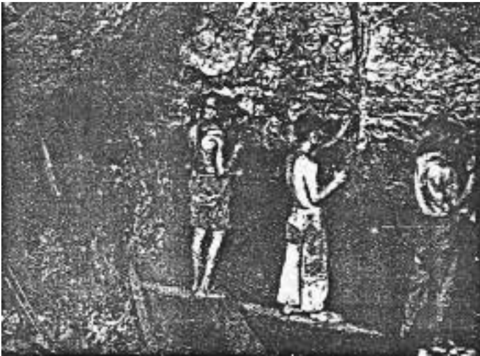
HAND DRILLING IN STOPE.
