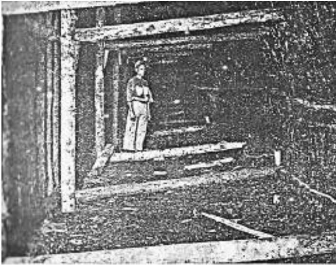
LONG WALL STOWAGE BARRICADE.
