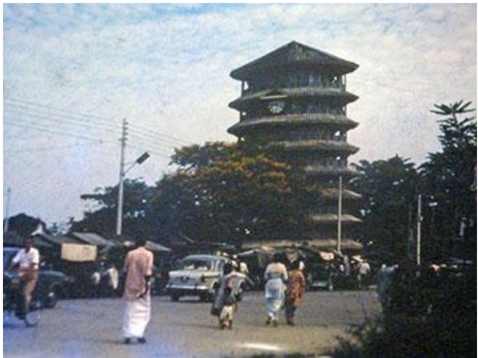
The Clock Tower in Teluk Anson Town Centre.
