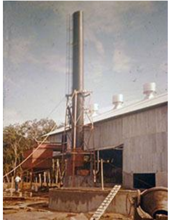
Selaba Factory being built.
