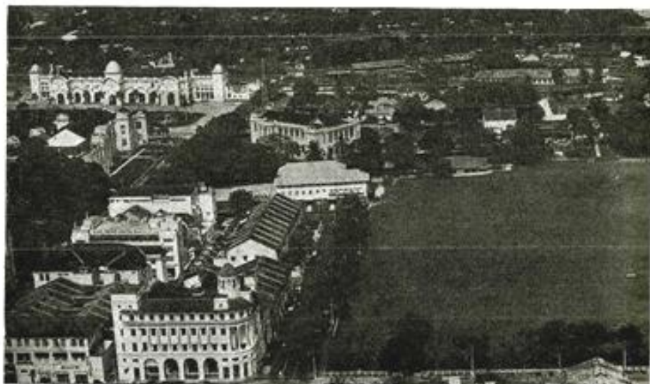
The heart of Ipoh. The Hongkong Bank building was a Japanese military office.
