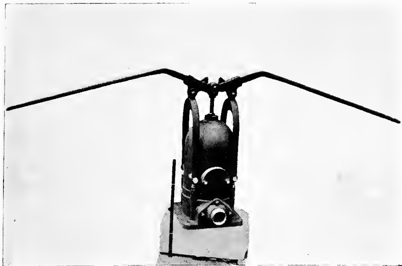
FIG. 2. THE FORCING "DANDO" PUMP.
