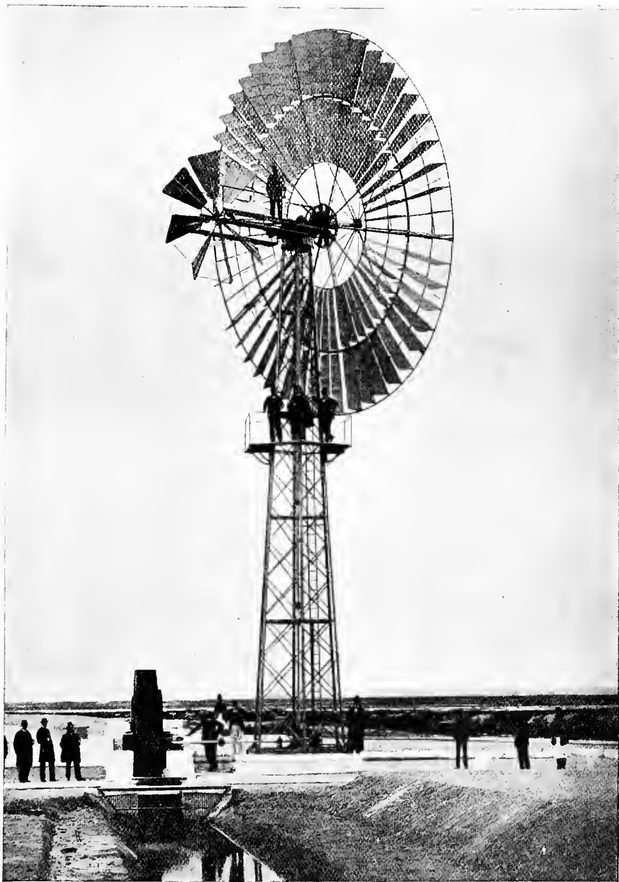
FIG. 13. LARGE PUMPING PLANT FOR RAISING SEA-WATER FOR DISTRIBUTION IN VAPORIZING BEDS FOR THE PRODUCTION OF SALT. DIAMETER OF WIND WHEEL, 37 FT. 6 IN.
