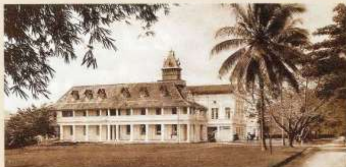
Batu Gajah courthouse built in 1892: The British headquarters of the Kinta region was moved to this town, 20km from Ipoh, in 1884
