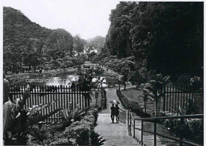
Figure 13. An abandoned tin-mining lake found its renewed purpose as a lake garden of Kek Lok Tong Cave Temple. (Ann 2012)
